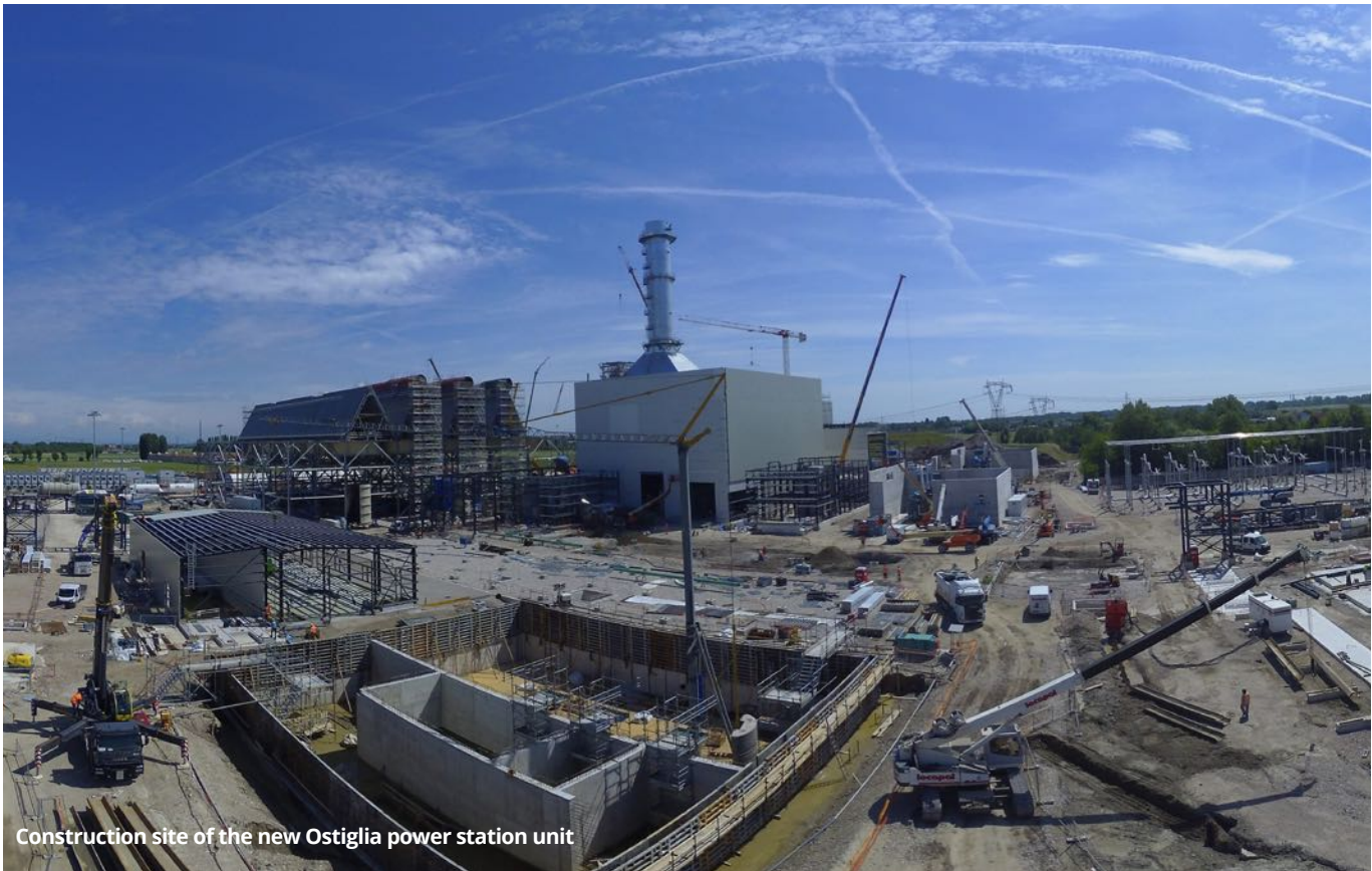
Construction site of the new Tavazzano and Montanaso power plant unit
